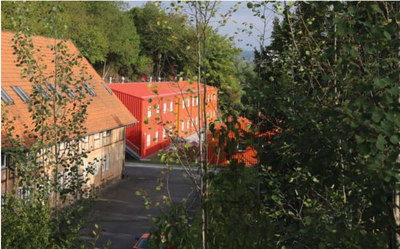
Refugee housing in Hünfeld / Photo: © Dr. Michael Fladung
