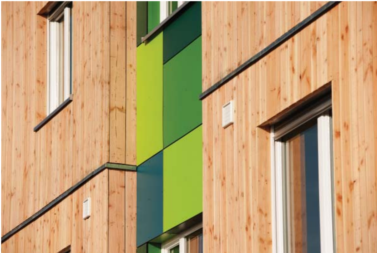
Detail facade / Photo: © Carsten Costard, Mainz
