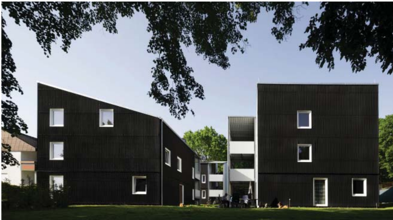
Exterior view / Photo © Markus Guhl
