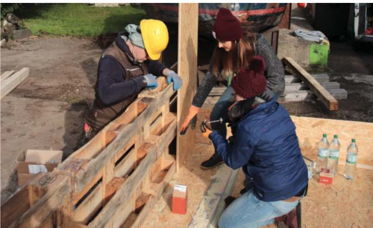
Construction / Photo: © Christian Hussong
