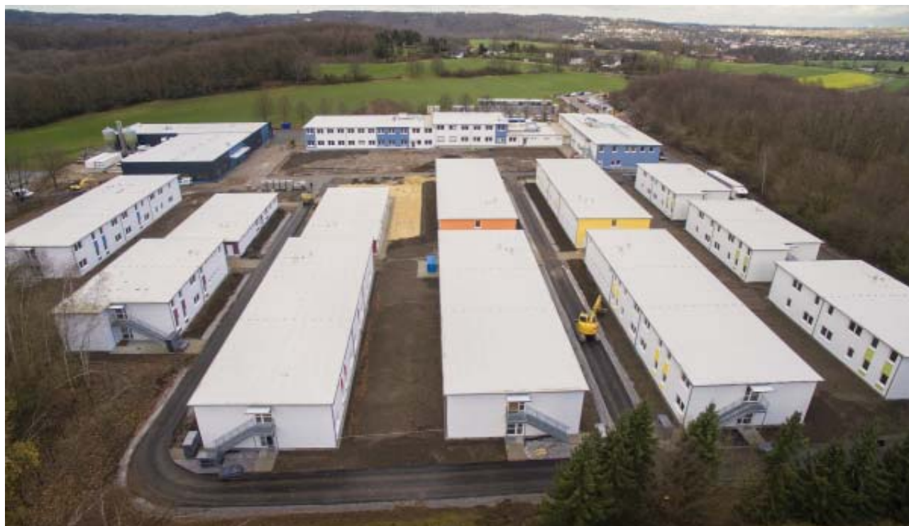
Aerial view / Photo: © GVE
