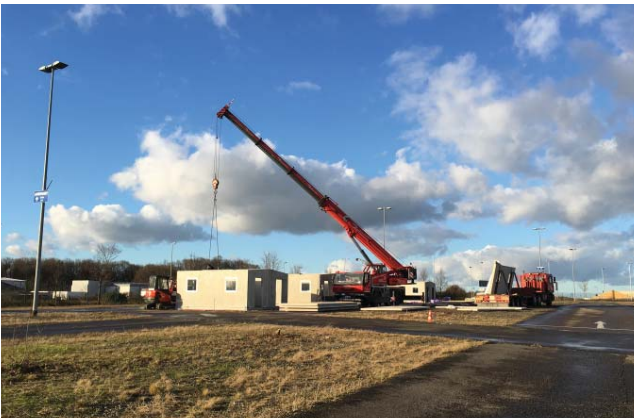
Construction site / Photo: © Martin Hachmeister
