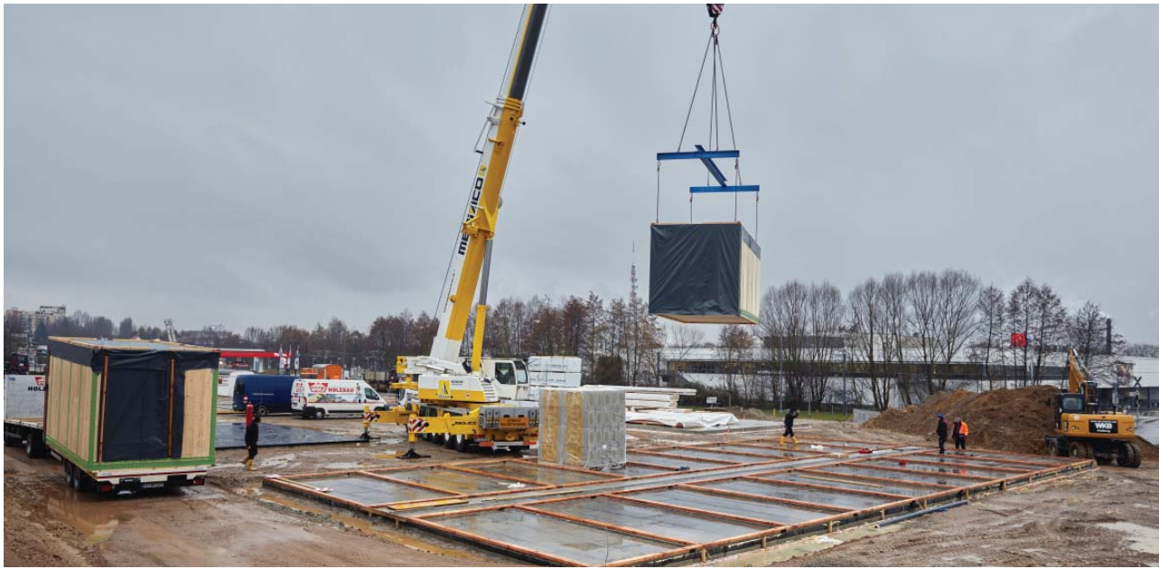
Gundelfinger street: Delivery of the modules / Photo: © Yohan Zerdoun
