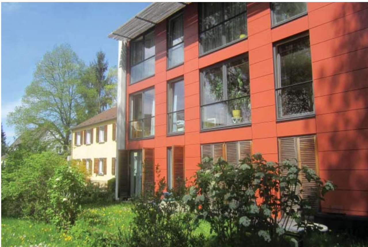
Europadorf: new building / Photo: © Thomas Körner-Wilsdorf
