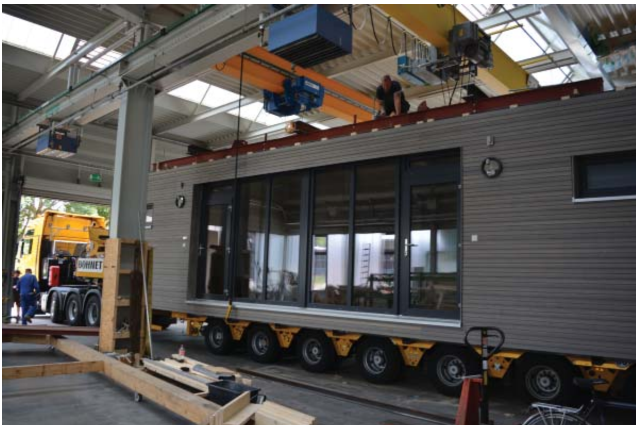
Producing the modules / Photo: © VARIAHOME
