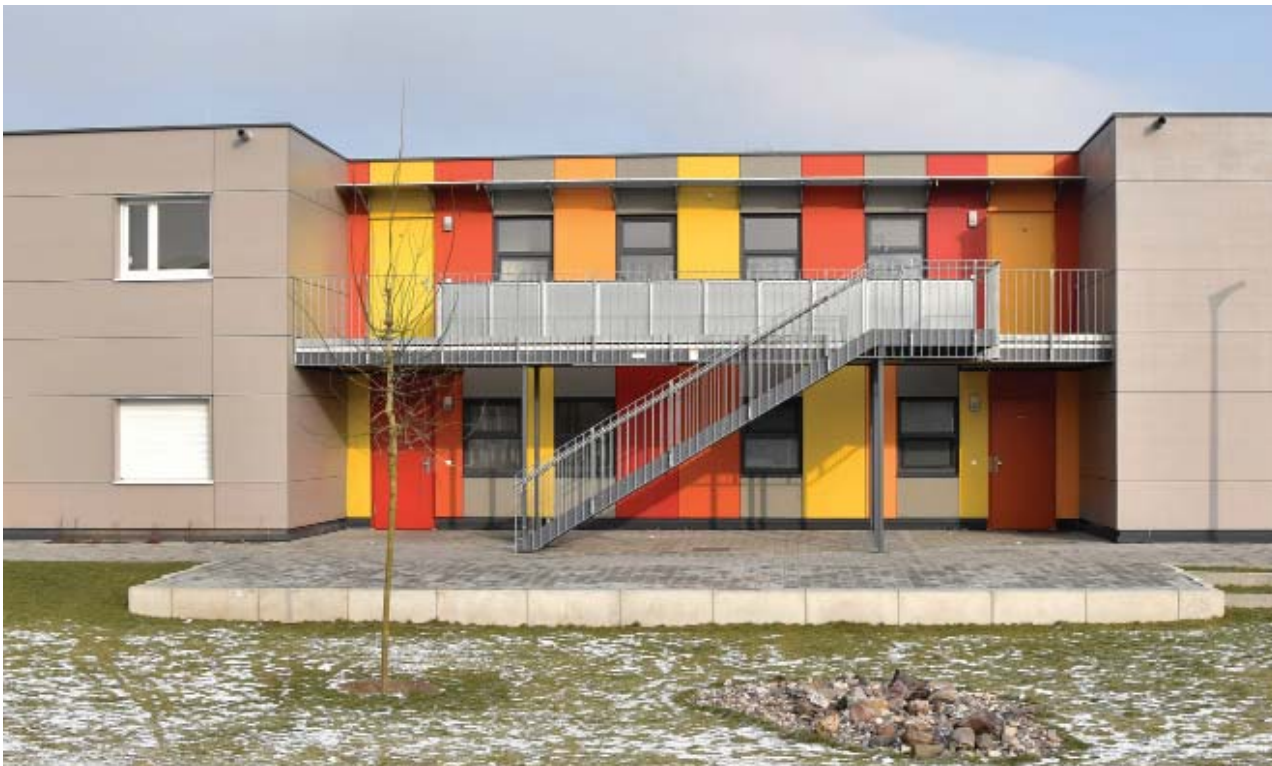
Corridor / Photo: © Olaf Rigoll
