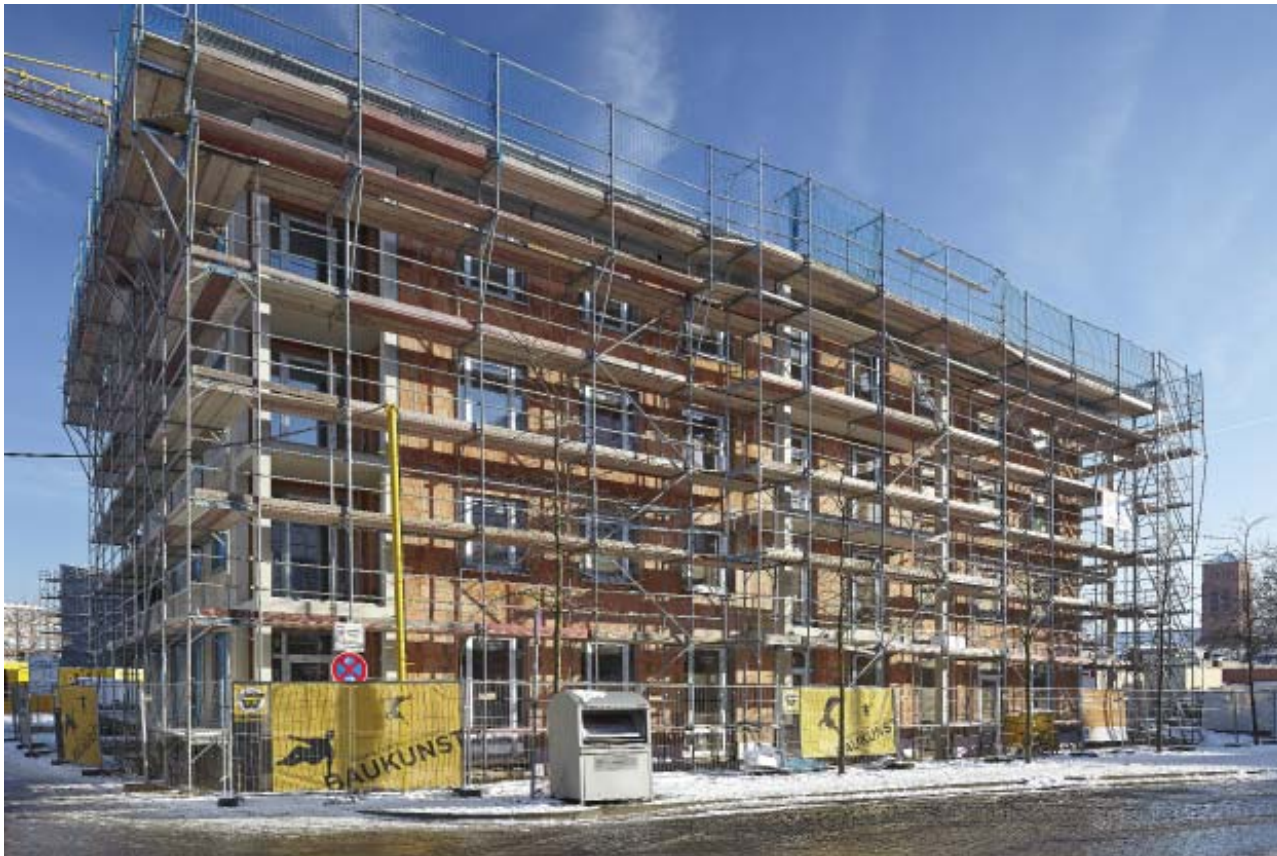
Construction site / Photo: © Wienerberger – Jens Krüger
