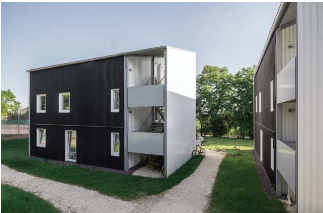
Exterior view / Photo © Markus Guhl
