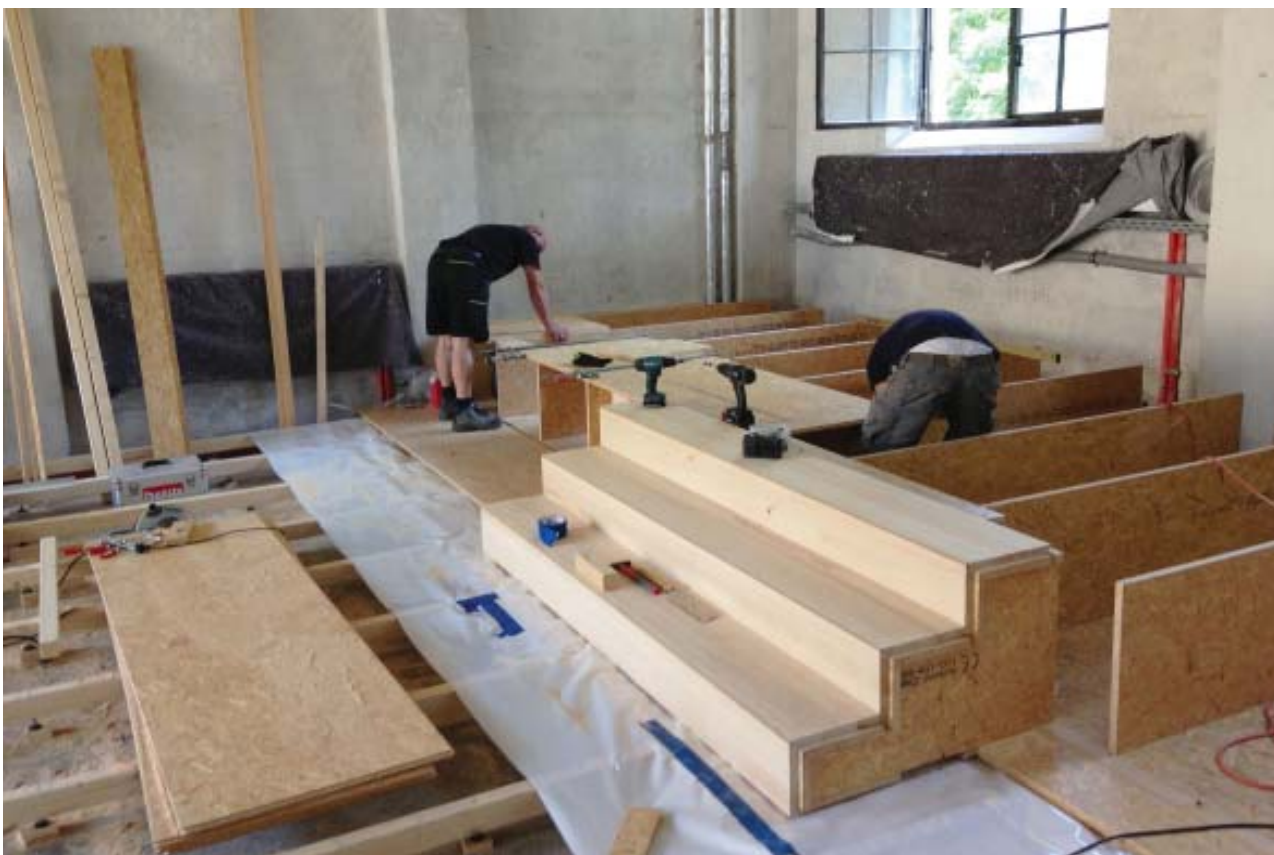
Construction site / Photo: © Thomas Körner-Wilsdorf
