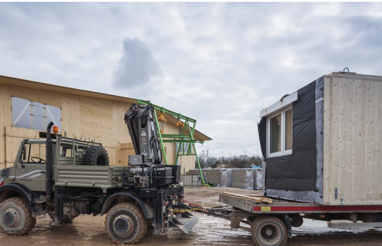
Transportation of room modules / Photo: © Michael Heinrich
