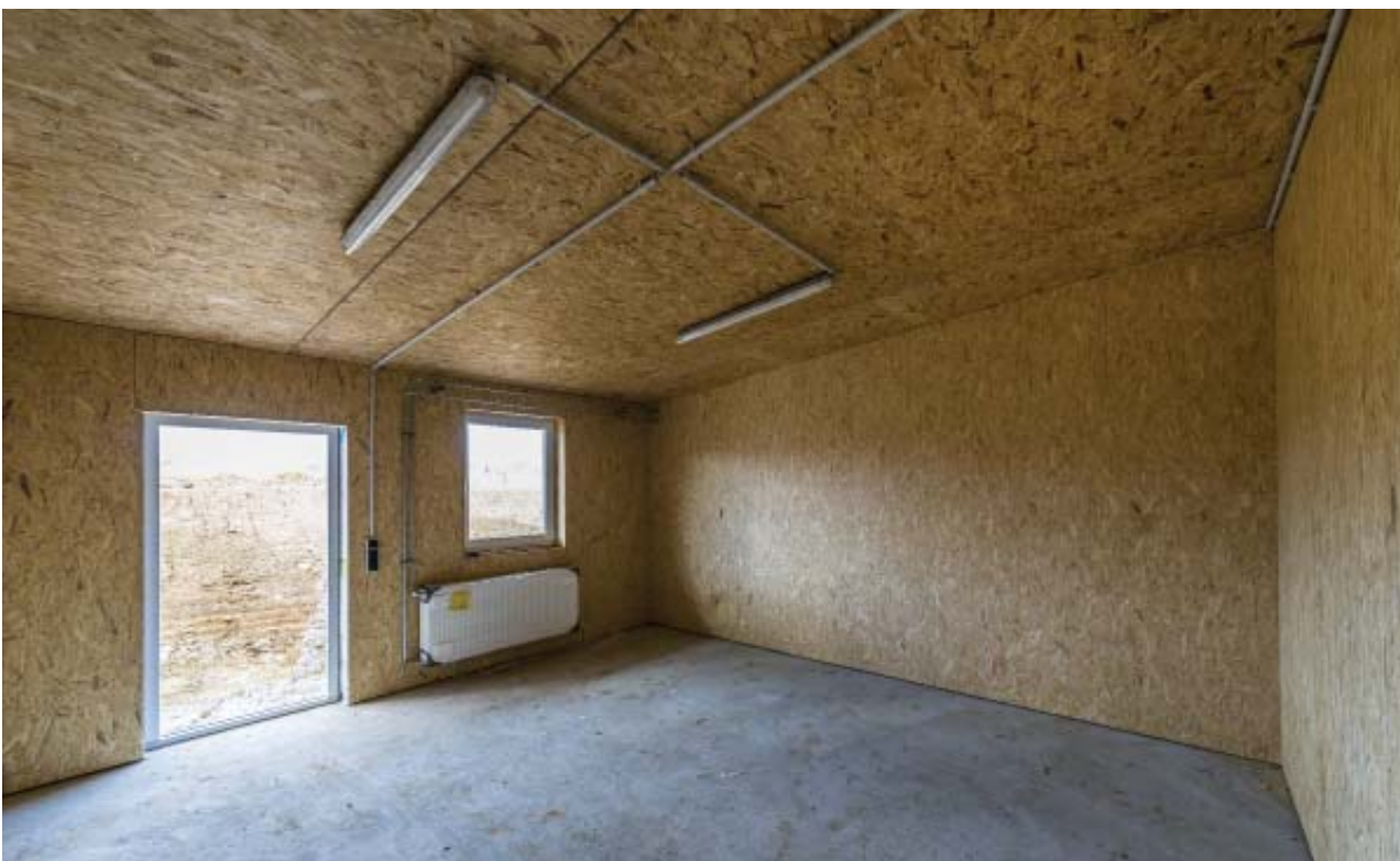
Interior / Photo: © Ulrich Schrader for Opitz Holzbau
