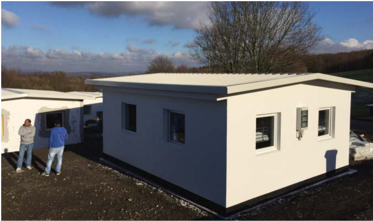
Construction site / Photo: © Martin Hachmeister
