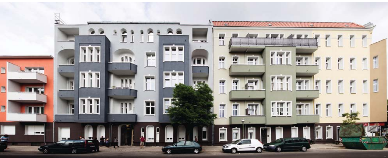
Building after renovation work / Photo: © Christian T. Joergensen
