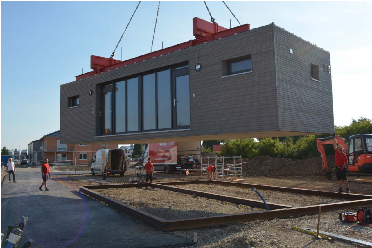
Königsbrunn: delivery of the modules / Photo: © VARIAHOME
