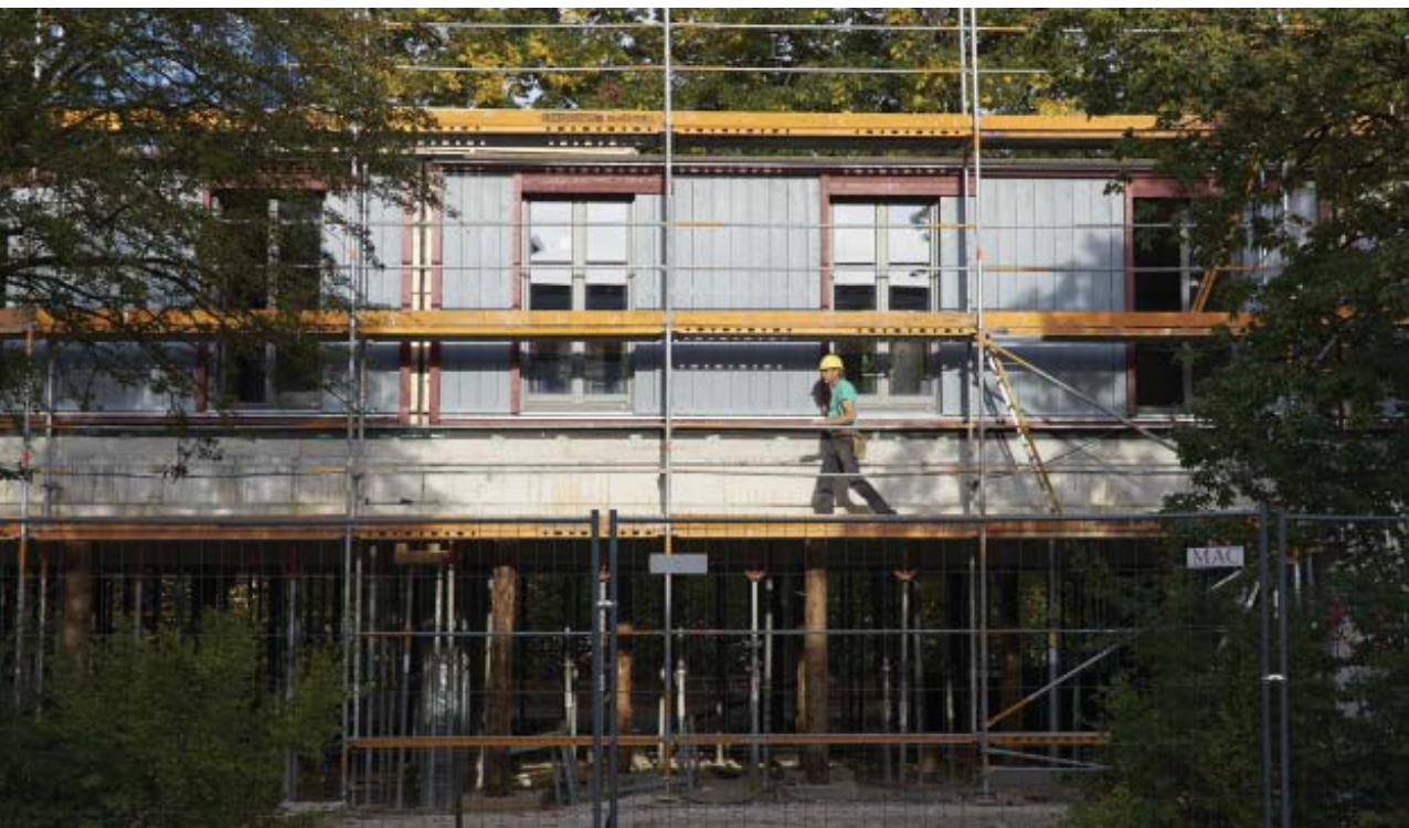
Construction site / Photo: © Stefan Müller-Naumann
