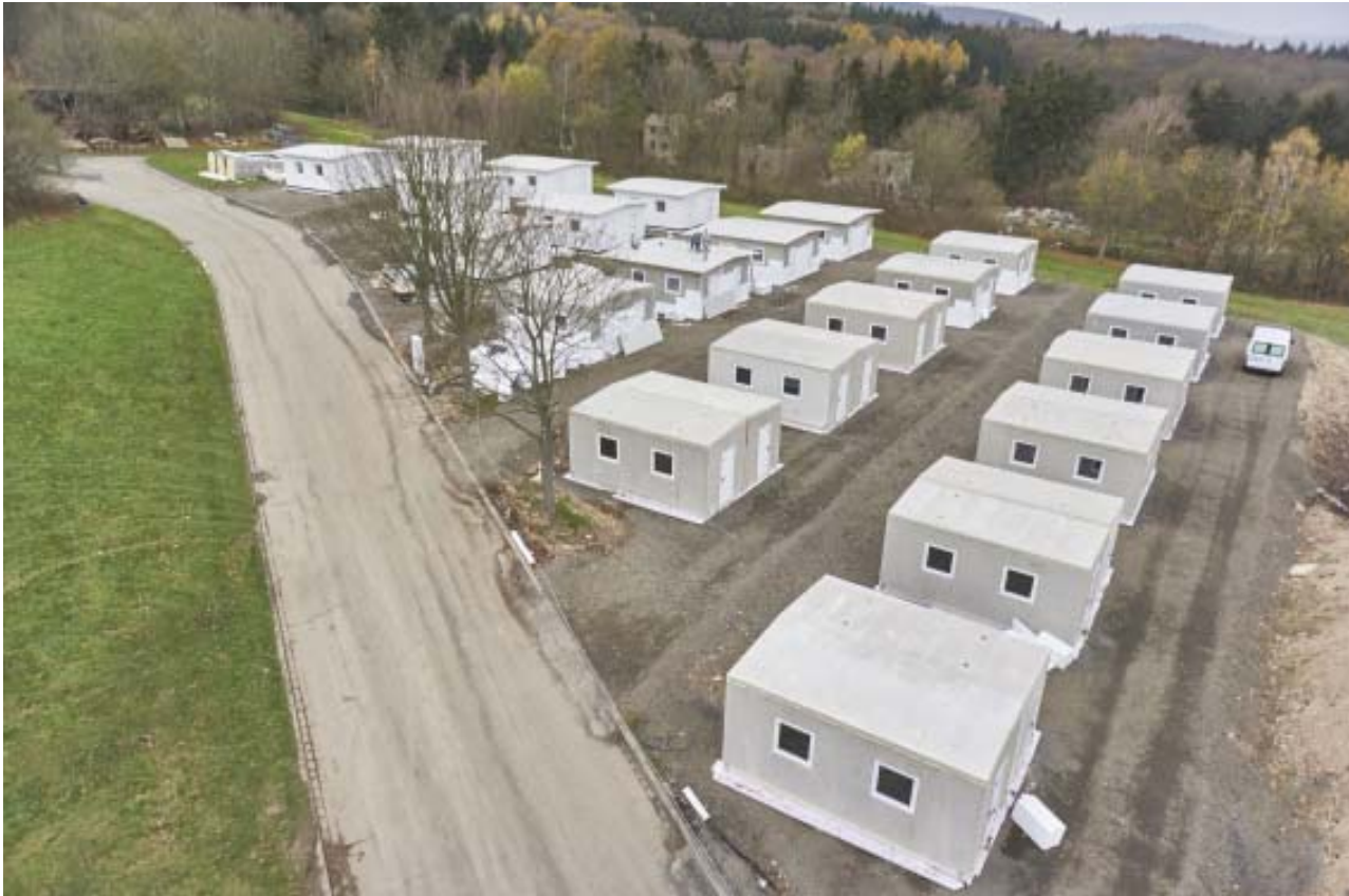
Aerial image / Photo: © OPTERRA / Sven-Erik Tornow
