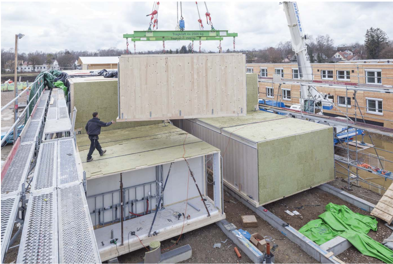
Assembly of room modules / Photo: © Michael Heinrich
