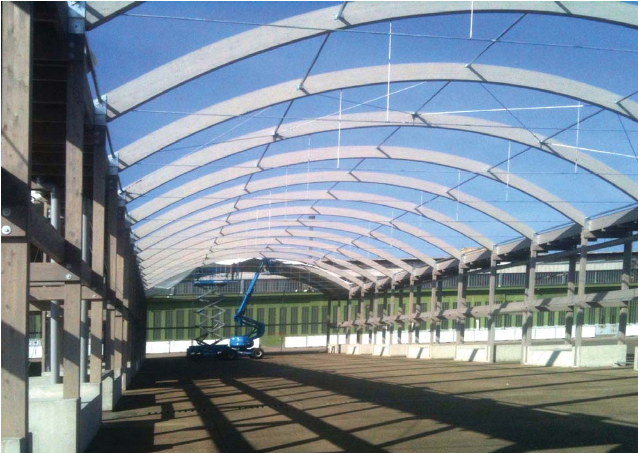
Constructing / Photo: © Gorenflos Architekten
