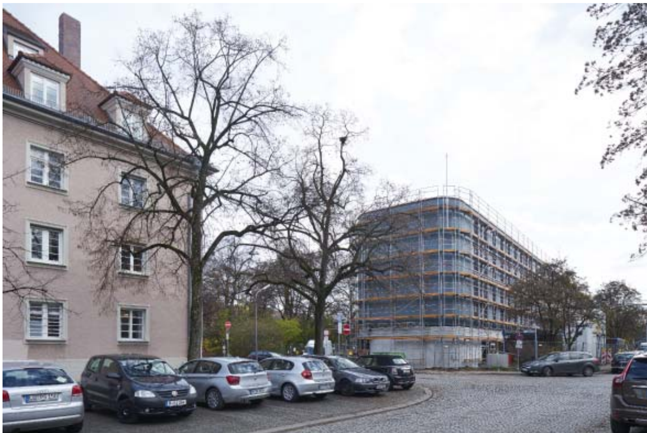
Construction site / Photo: © Stefan Müller-Naumann
