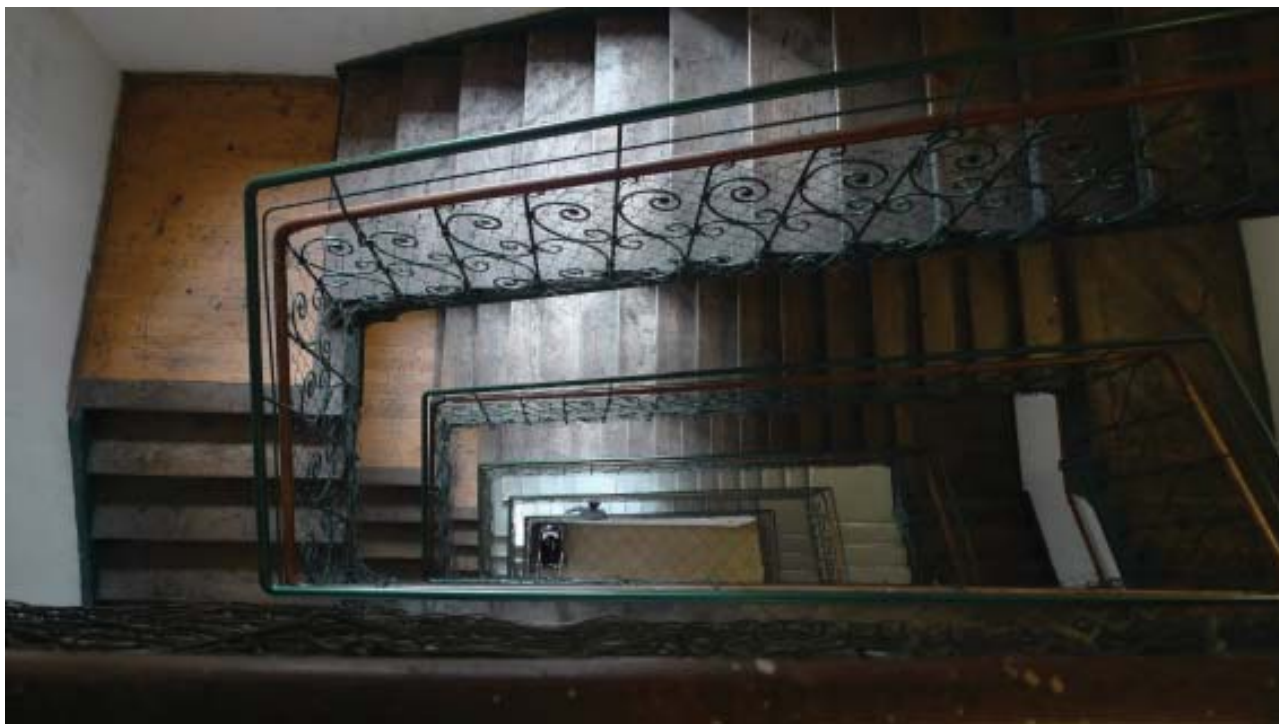
Stairwell / Photo: © Nele Bayer
