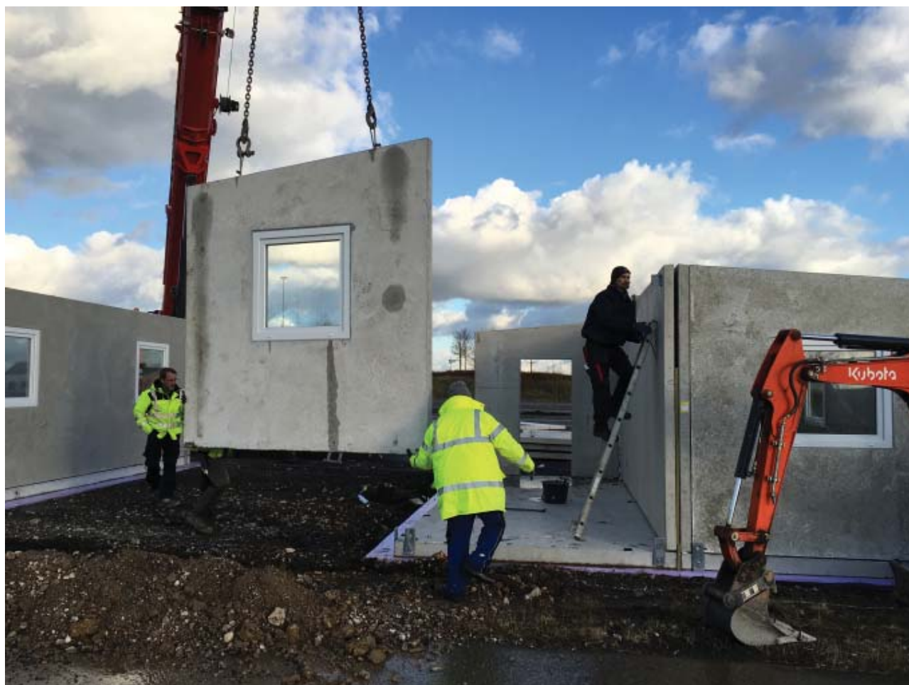
Construction site / Photo: © Martin Hachmeister
