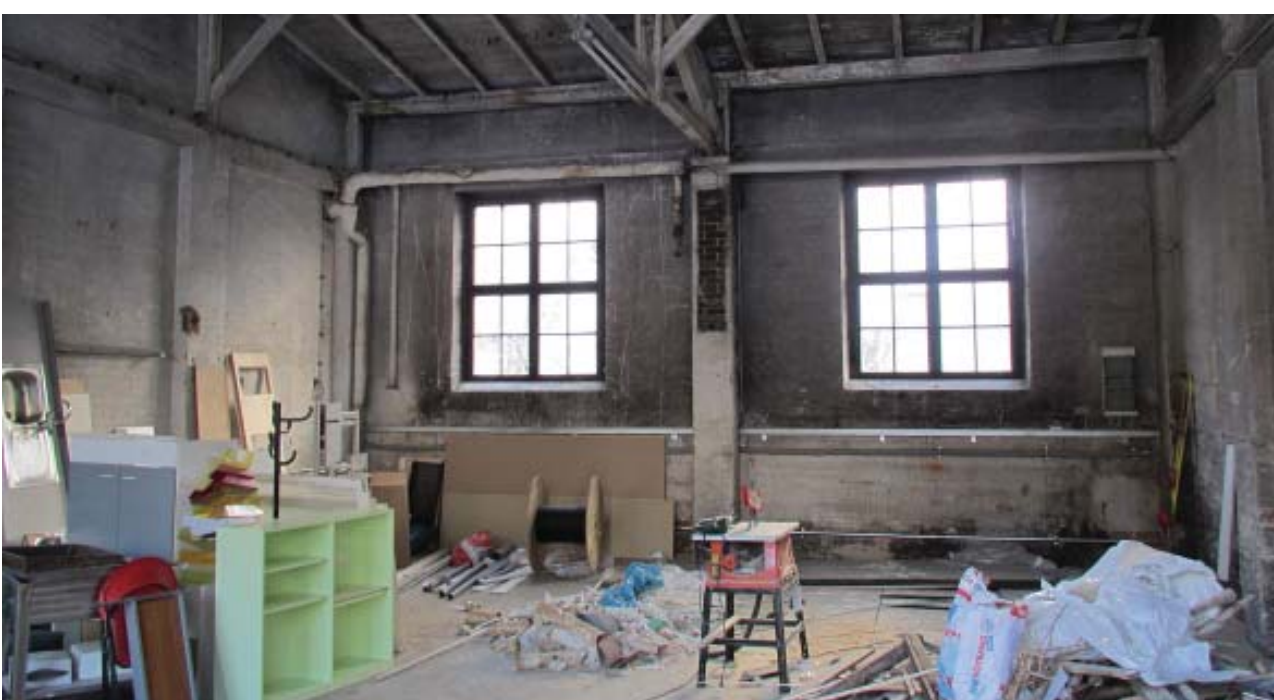
Construction site / Photo: © Thomas Körner-Wilsdorf
