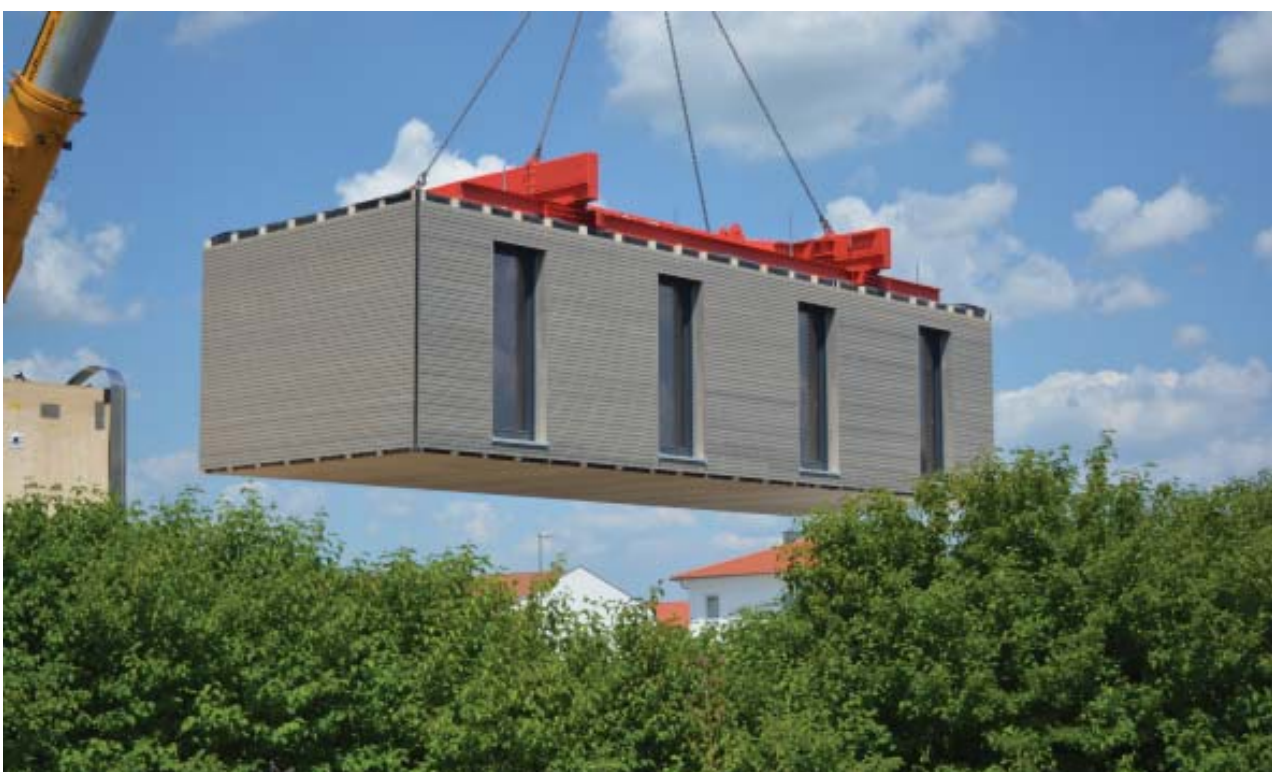
Königsbrunn: Delivery of the modules / Photo: © VARIAHOME
