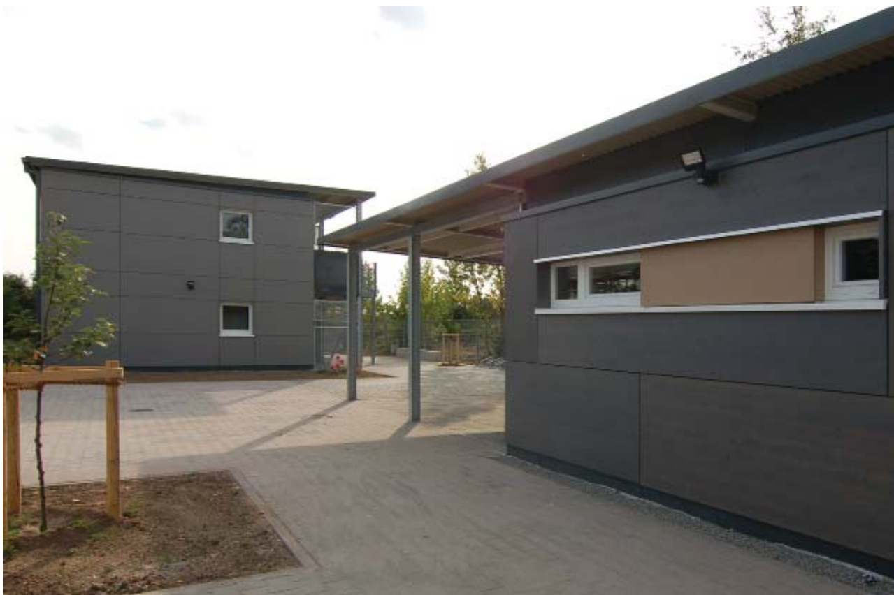
Flörsheim am Main: community building / Photo: © Olaf Rigoll
