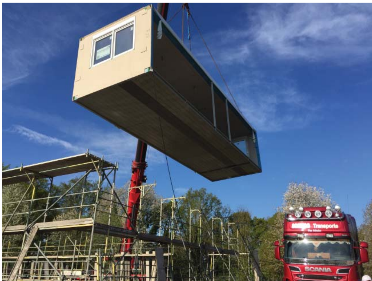
Delivery of the first modules on 28 Apr 2015 / Photo: © GVE
