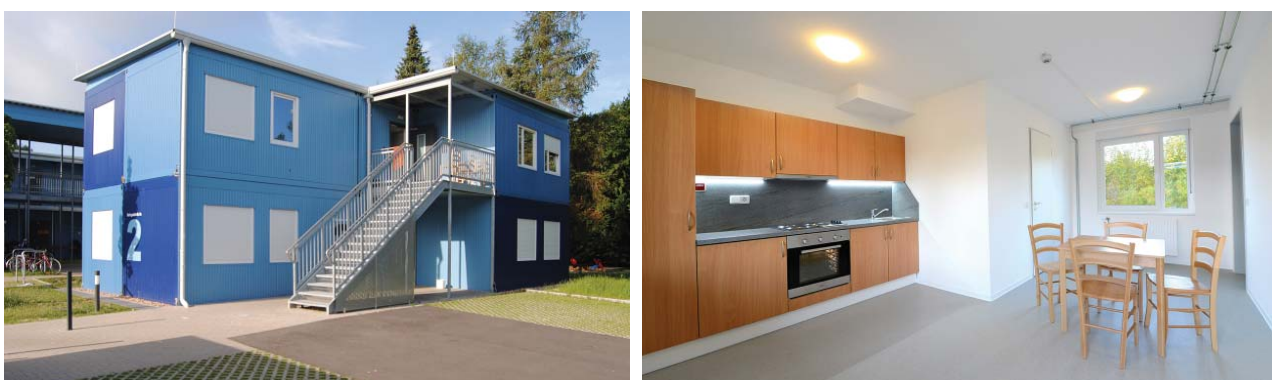
Grohn: Containers and interior / Photo: © Feldschnieders + Kister Architekten
