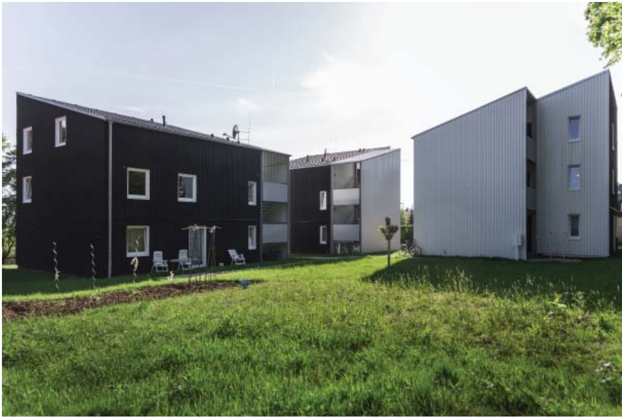
Exterior view / Photo © Markus Guhl
