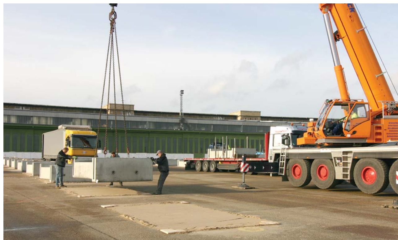
Constructing the foundations / Photo: © Gorenflos Architekten
