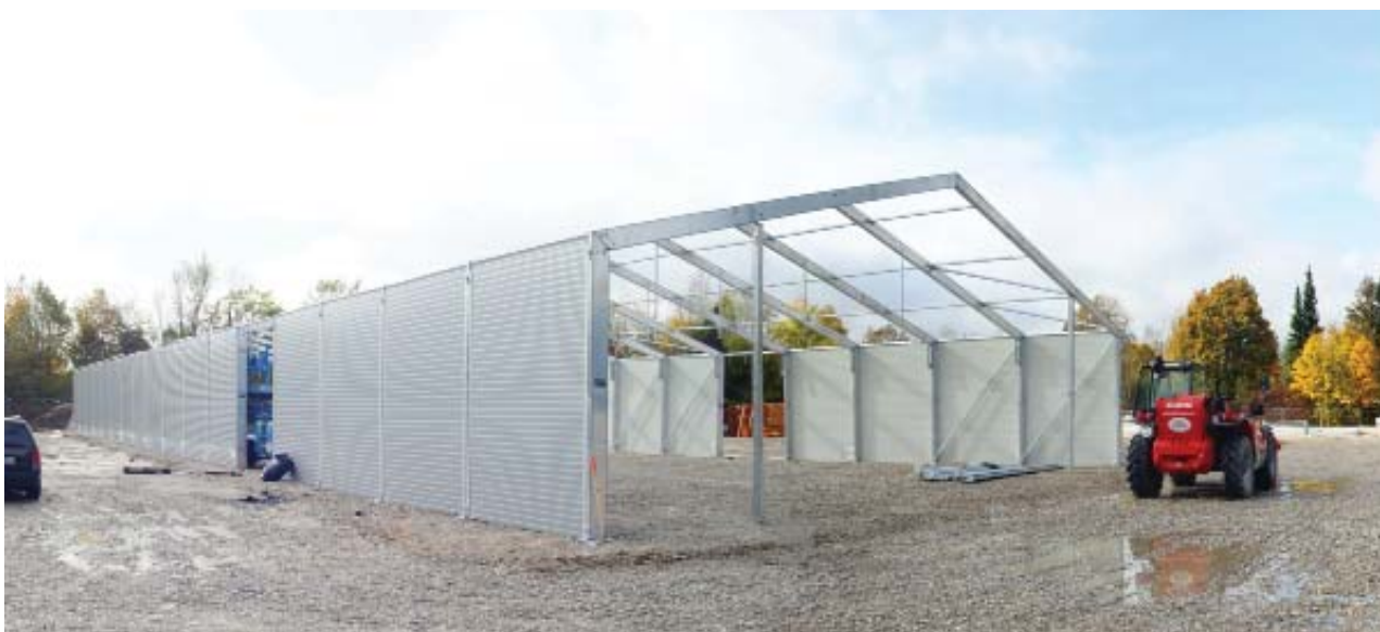
Construction of light-frame hall / Photo: © Jan Schabert
